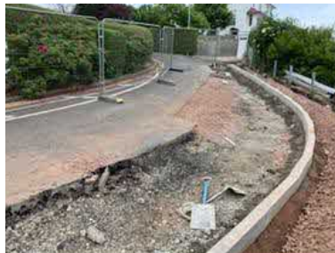
Road being prepared for re tarmacing
