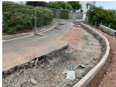
Road being prepared for re tarmacing
