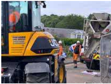
Gabions being installed adjacent to proposed development site
